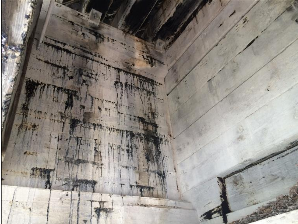
Photo #19 Abutment 2 interior face of Girder 2
