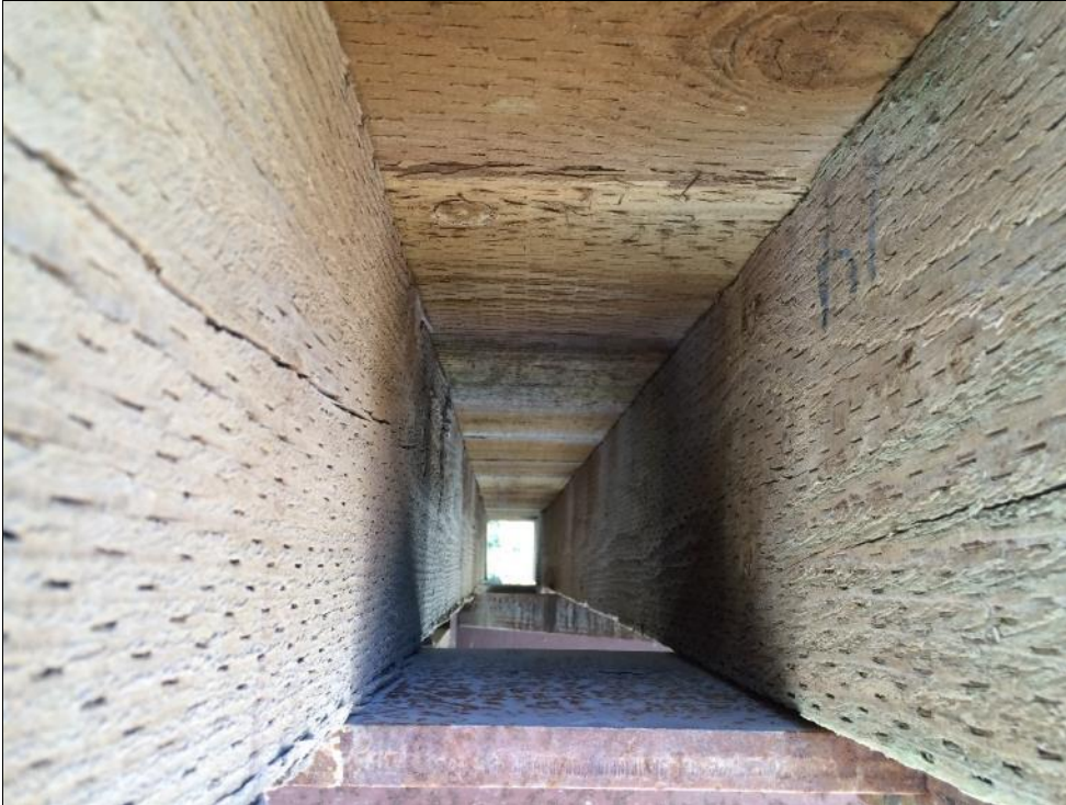
Photo #29 Span 1 (new) deck structure looking between transverse ties
