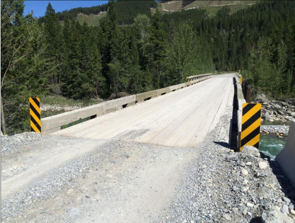
Photo #3 Abutment 1 approach
