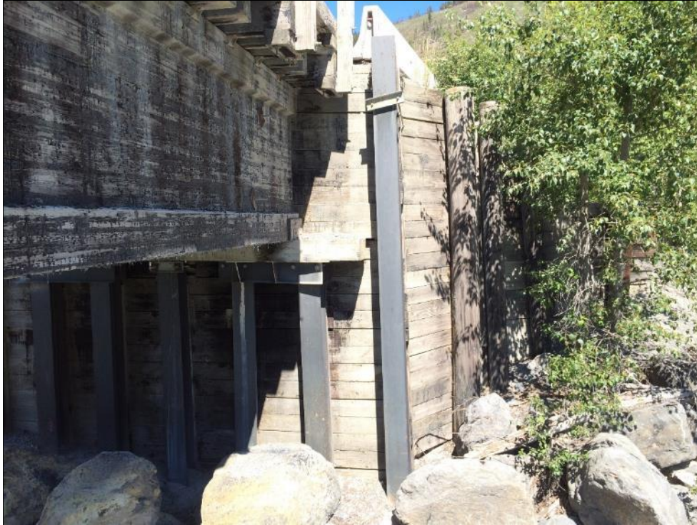
Photo #17 Abutment 2 U.S side
