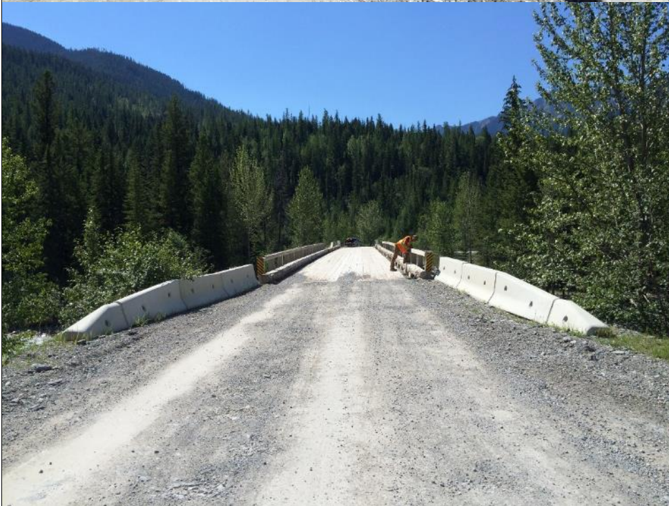
Photo #4 Abutment 2 approach
