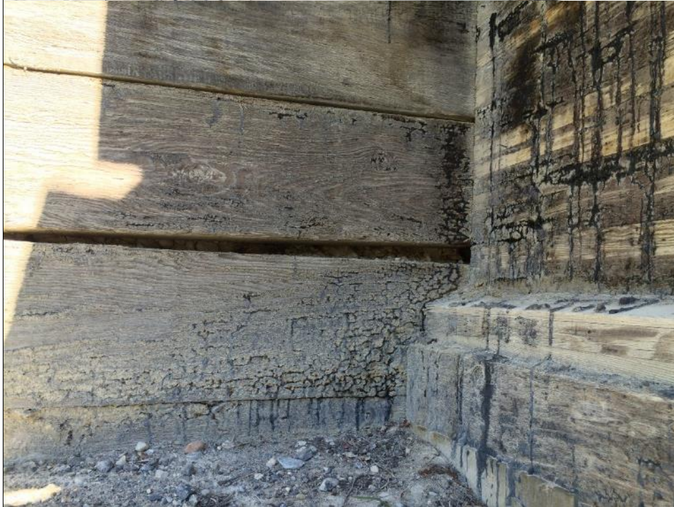
Photo #20 Abutment 2 D.S. end of Girder 2 / ballast wall
