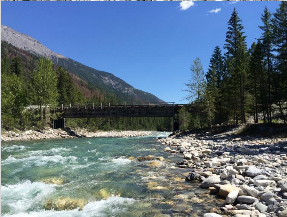
Photo #2 Downstream elevation
