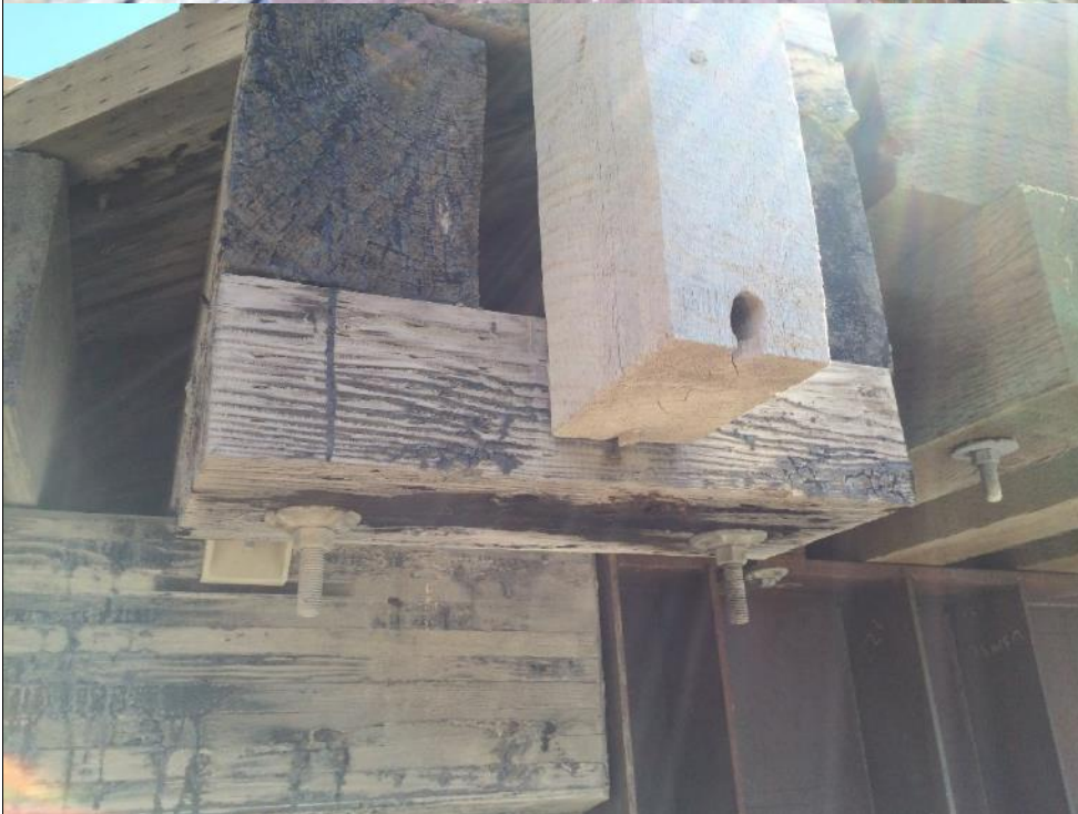
Photo #30 Span 2 (old) deck structure
