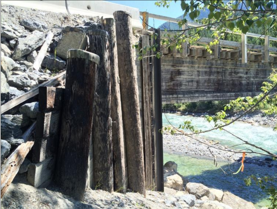
Photo #21 Abutment 2 D.S wingwall
