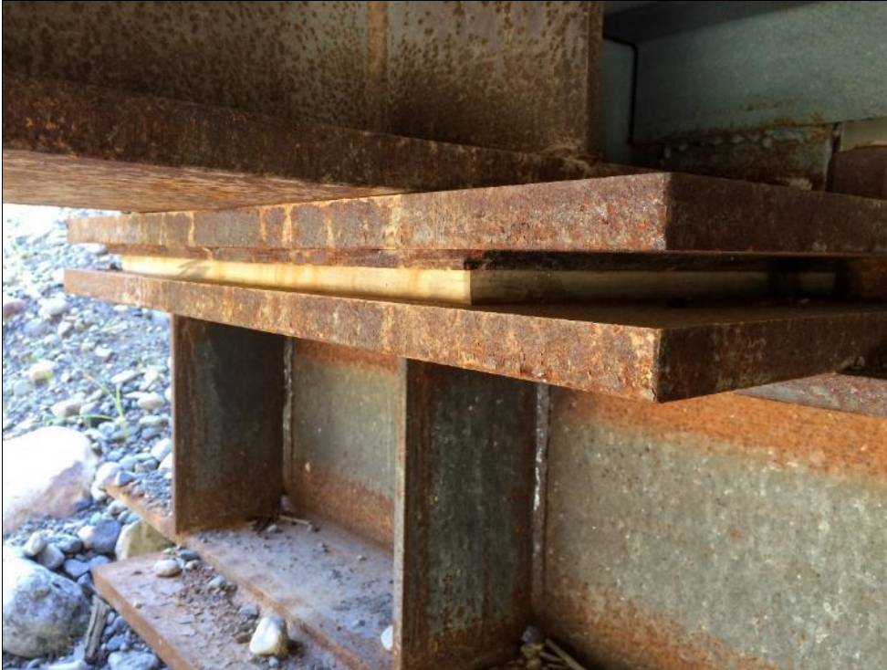
Photo #7 Abutment 1 U.S bearing
