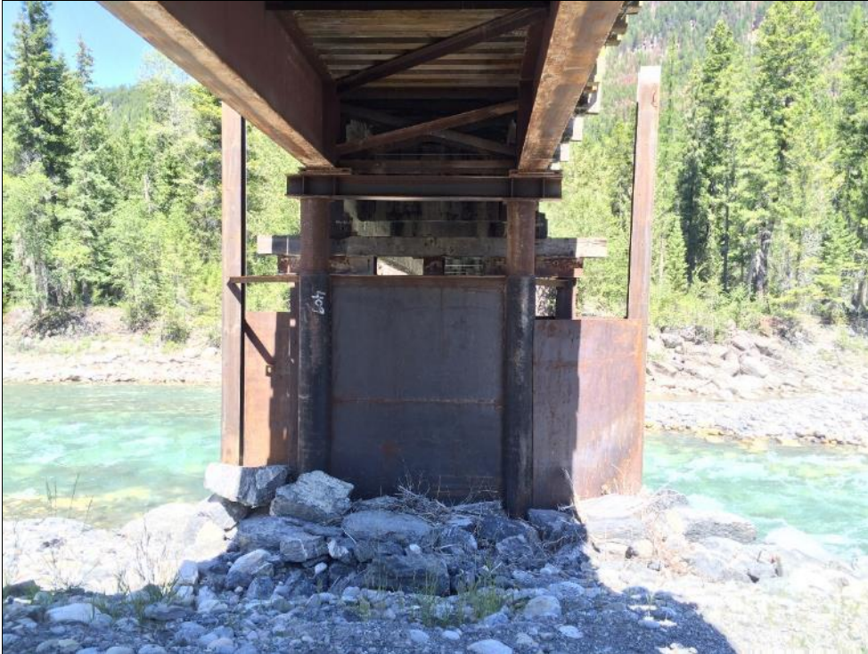
Photo #15 Pier 1 looking to Abutment 2
