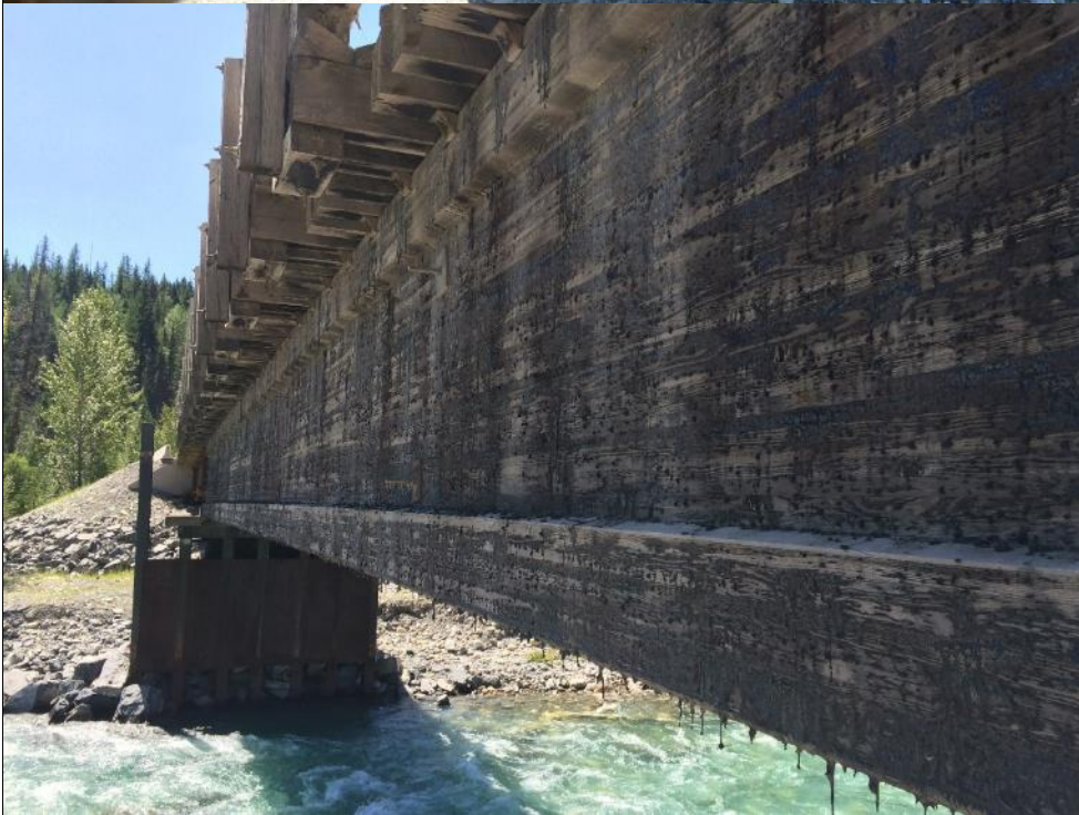
Photo #24 Span 2, Girder 1 looking to Abutment 1
