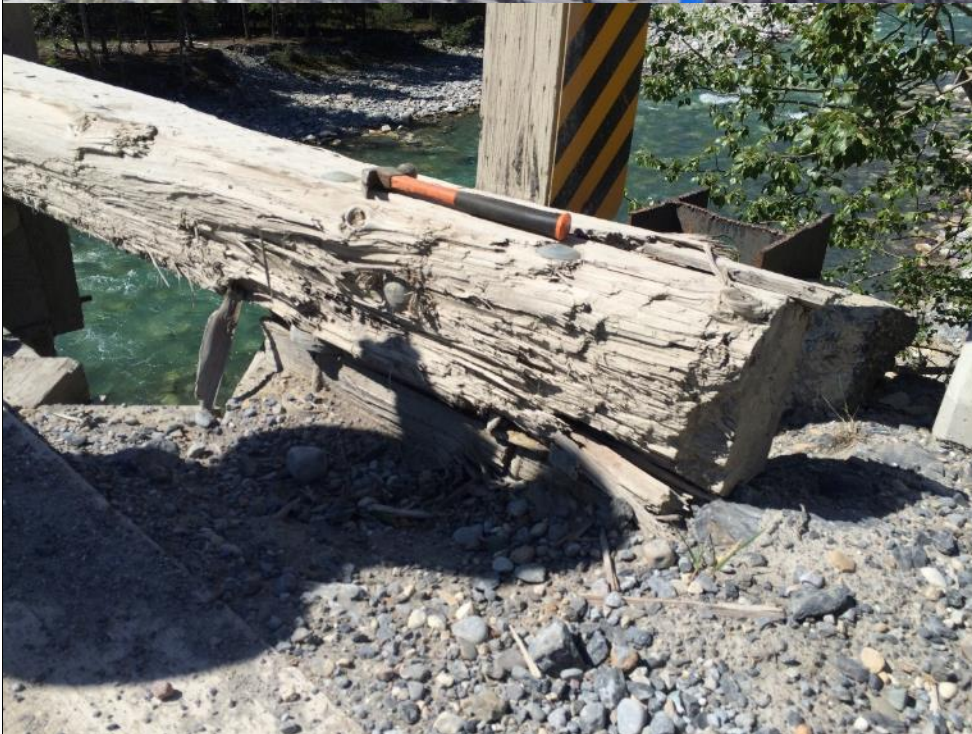
Photo #28 End of curb rail at Abutment 1
