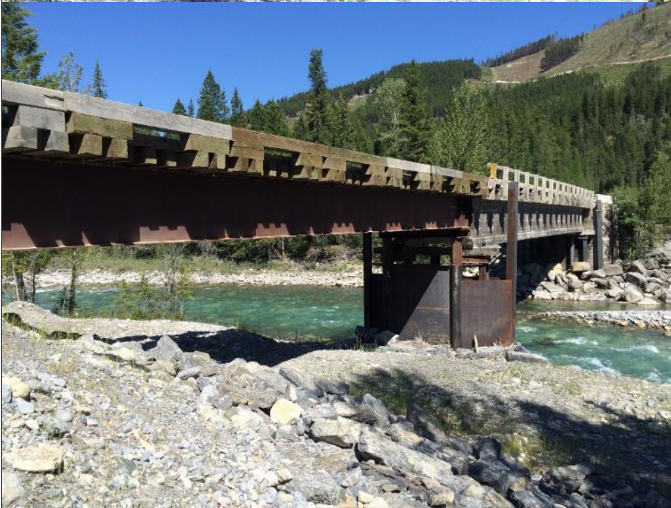
Photo #22 U.S / Girder 1 elevation looking to Abutment 2
