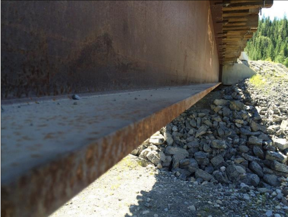
Photo #23 Span 1, Girder 2 looking to Abutment 1
