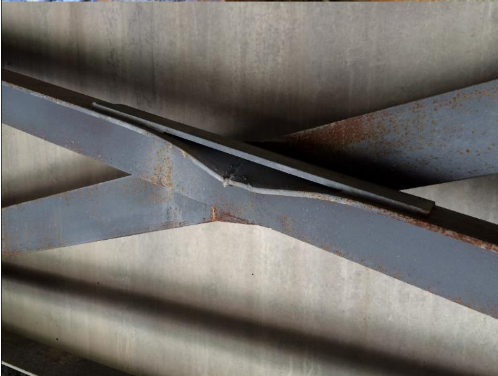
Photo #8 Abutment 1 steel diaphragm
