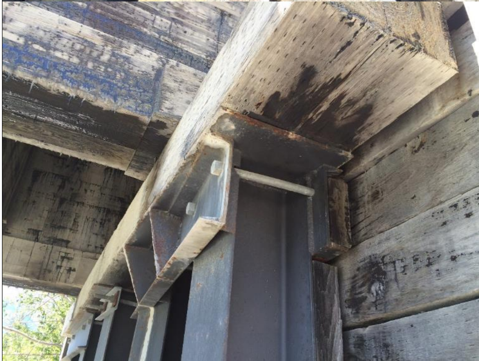
Photo #18 Abutment 2 U.S end of cap
